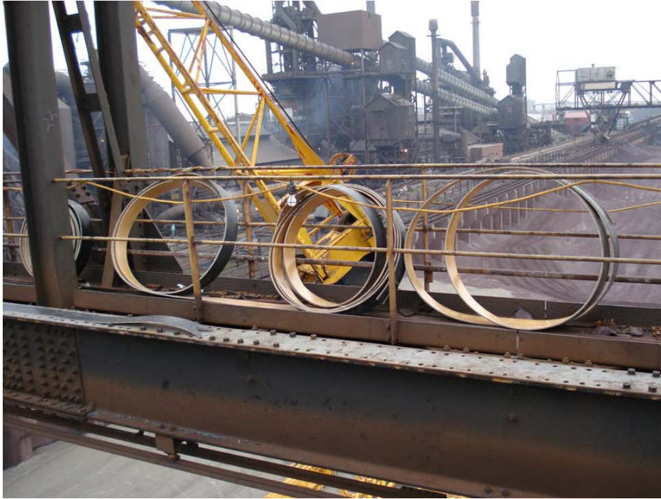
The ore bridge is 600' long and used 1200' of Fabreeka-LTP pad.
