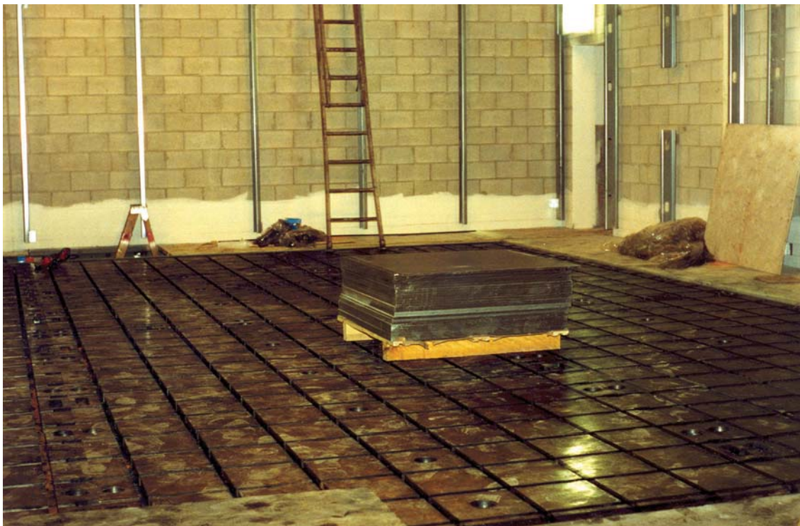
Finished mass with bed plate. The bed plate weighs an additional 85,000 lbs.
