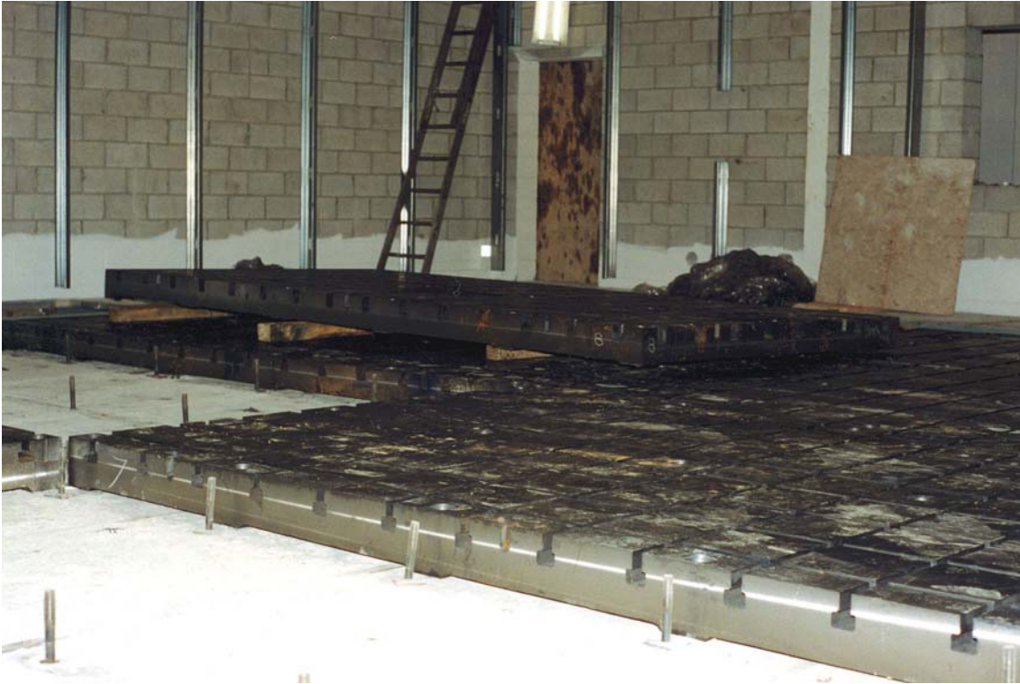
Installing and levelling the bed plate on the anchor bolts. The dynamometers will be installed on the bed plate and will weigh over 40,000 lbs.
