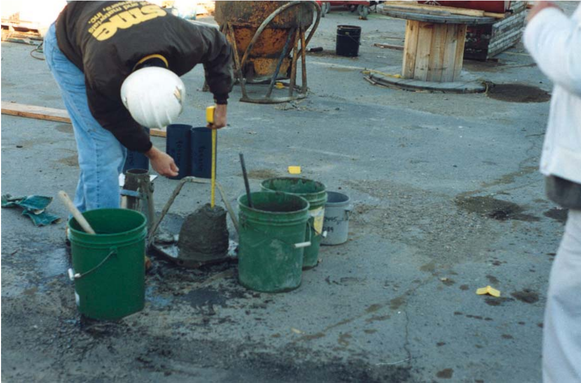
Concrete sample testing during the mass pour.
