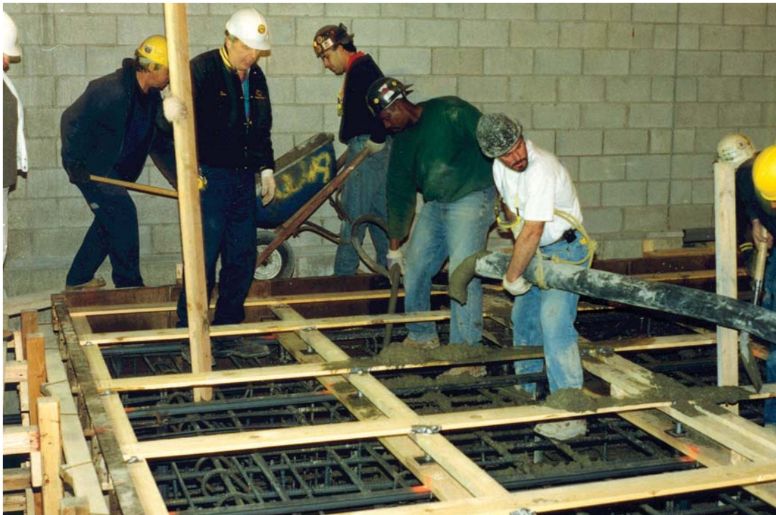
Concrete pour. The mass will weigh approximately 720,000 lbs without bed plate or dynamometers installed.
